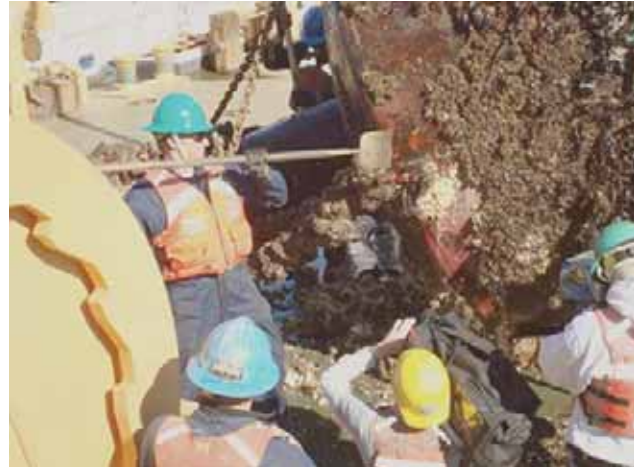
Figure 709. USCG removing marine growth from a buoy.
