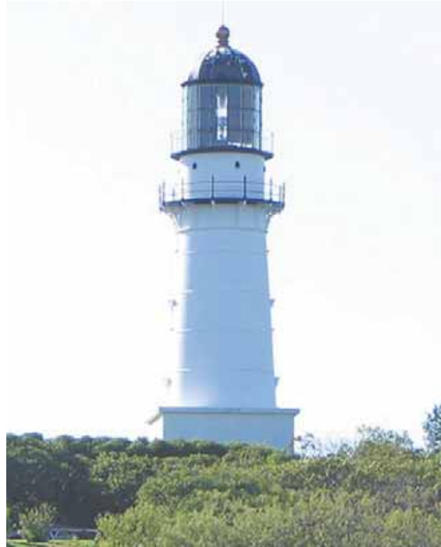
Figure 712. Typical Major Light.
