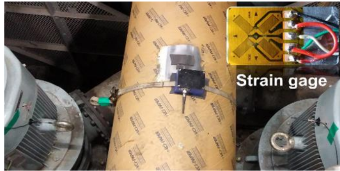
Figure 3 Telemetric system and strain gage installation
