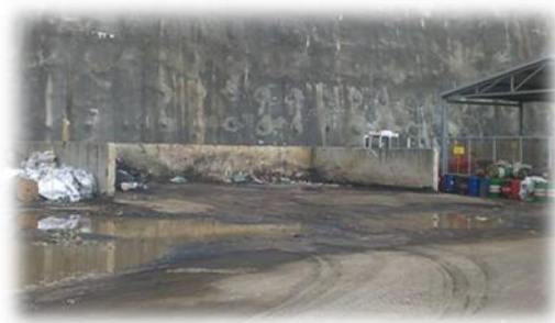
Figure 2 Landfill for temporary sediment disposal
